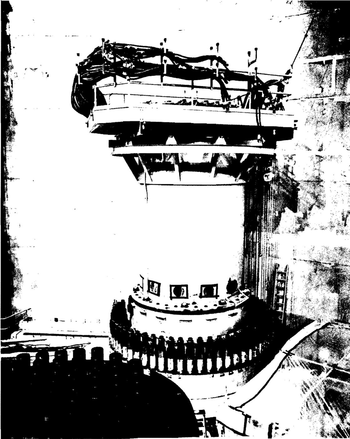
Figure 5. TMI-2 reactor head service structure.
